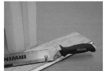
Lay the rest, plank after plank, in this manner until you have completed the first row. Cut the last plank accordingly. Ensure that this first row is straight using the wedges to maintain proper 3/8" expansion space from the wall. Planks may require scribing and cutting to fit wall curvature if present.
